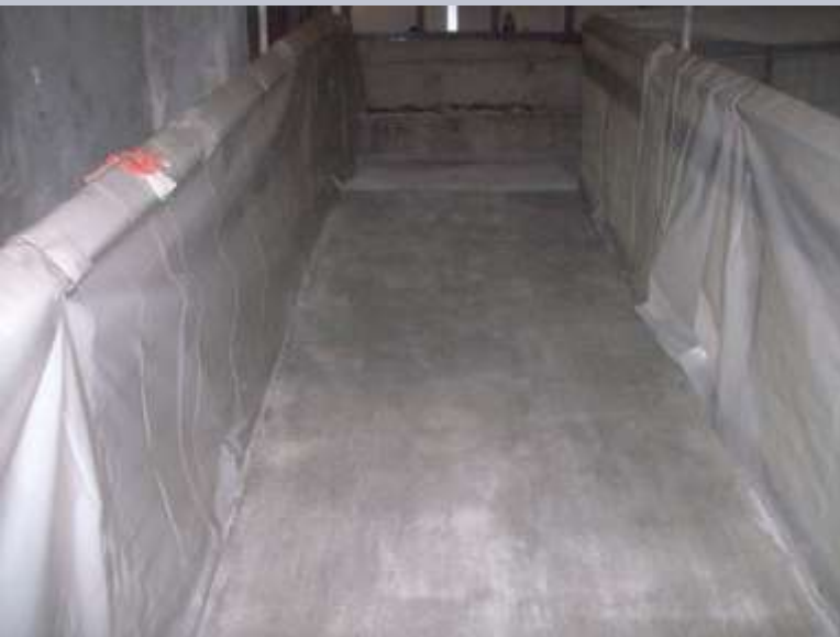
RAMP AFTER CONCRETE PLACEMENT
