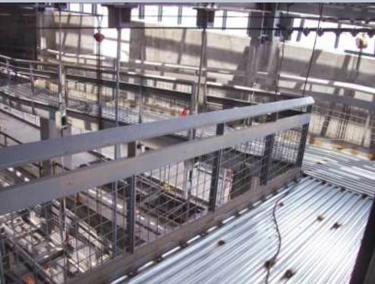
METAL DECK AND GUARD RAIL
