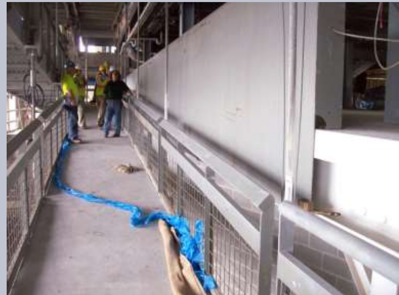
RAMP AFTER CONCRETE PLACEMENT
