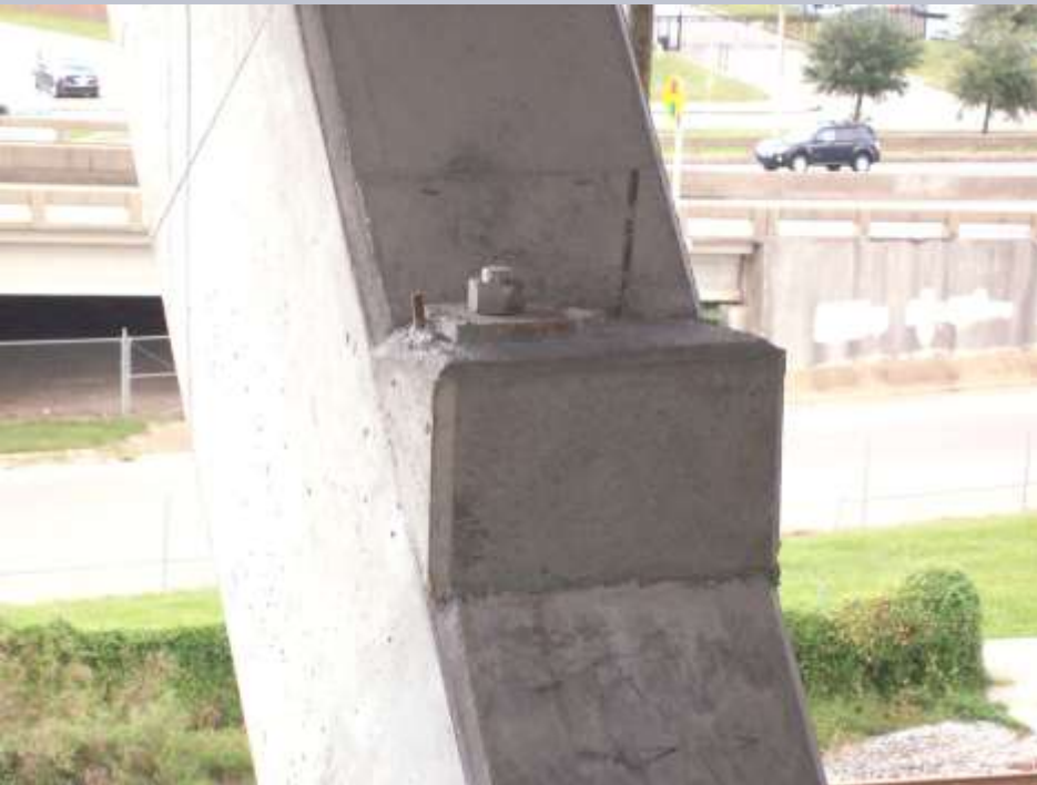
HOLES OMITTED – SOME RAKERS WERE DRILLED FOR ROD
