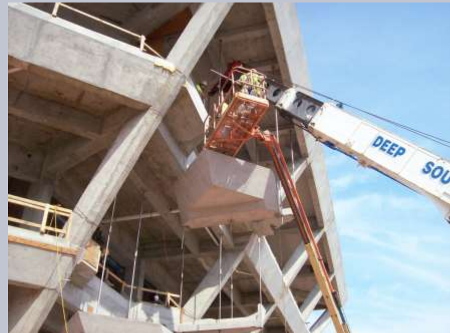
STAIR LANDING ERECTION
