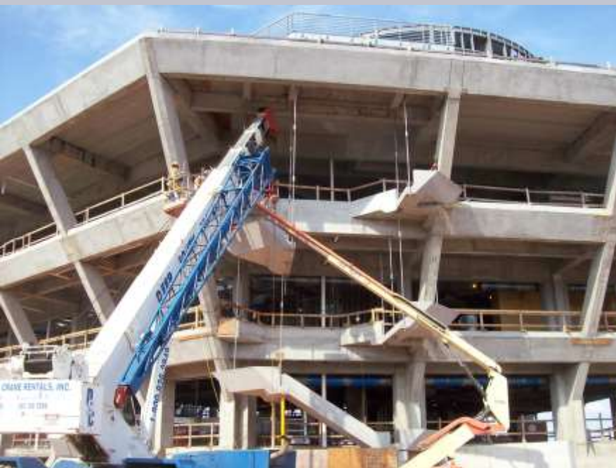
STAIR LANDING ERECTION
