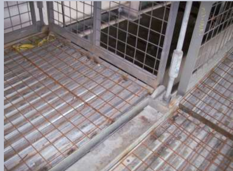
METAL DECK AND GUARD RAIL
