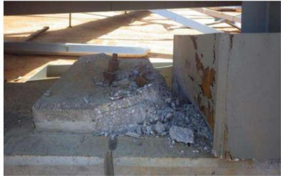
Photograph 19: The majority of the concrete pile caps are cracked.
