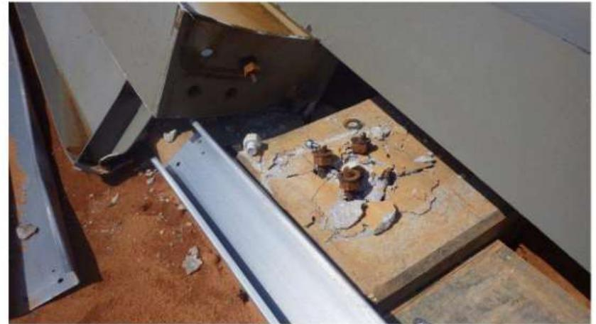
Photograph 18: The majority of the anchor bolts are sheared, either above or below the base plate of the rigid frame columns.
