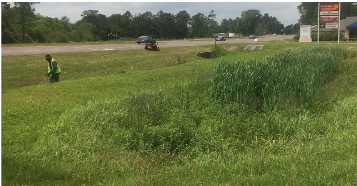
Stormwater conveyance and detention basin maintenance. (Photo courtesy of Barry Fagan.)
