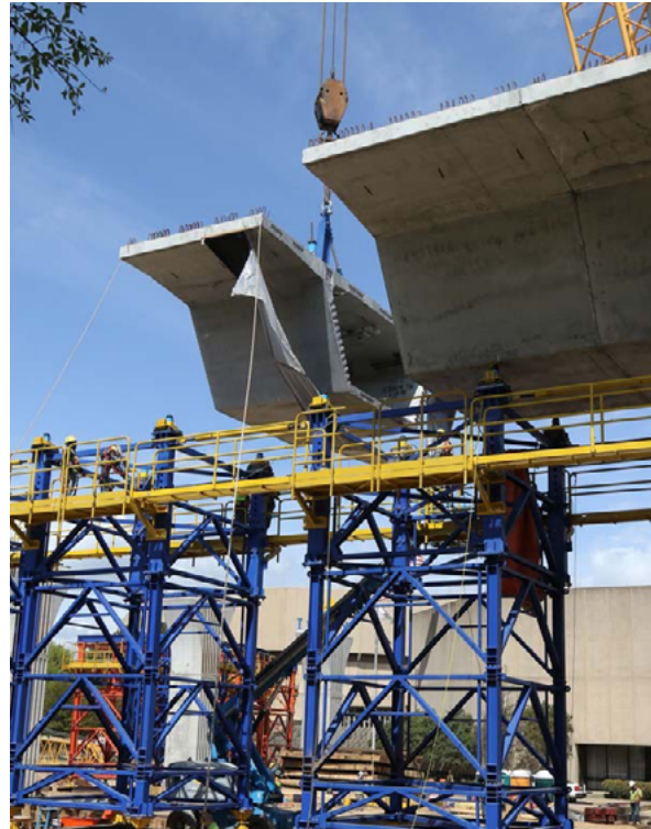
Concrete segment erection on CBD mainline bridge on I-20/59.
