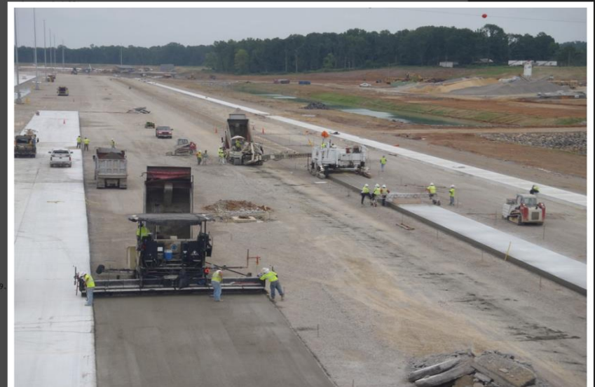
RCC and PCC Installation Image 1 of 3
