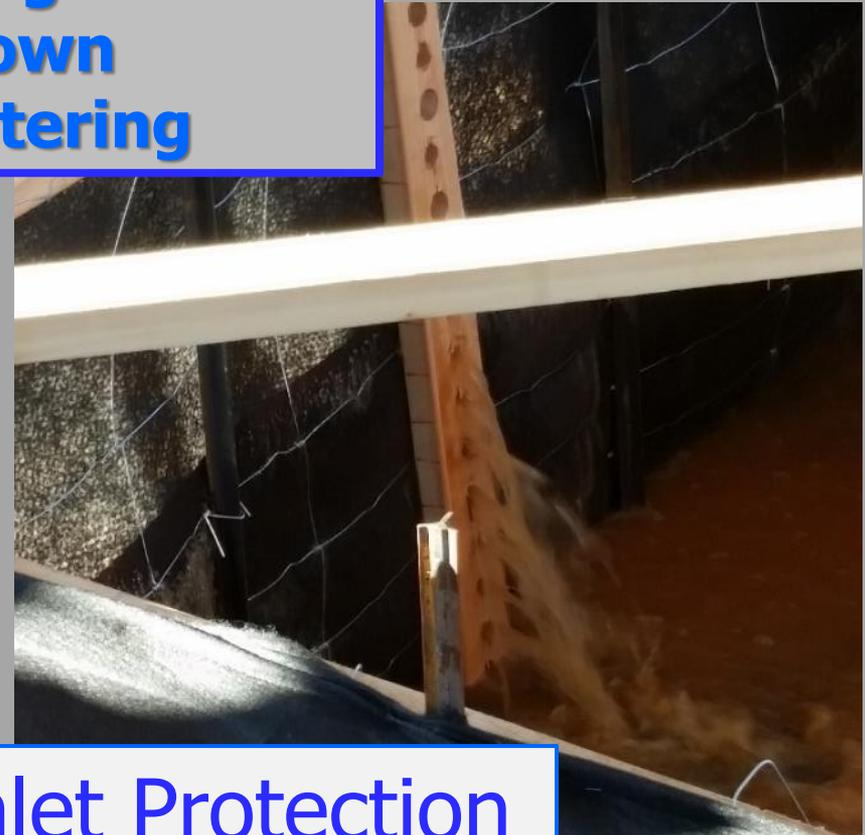
**Silt Fence Inlet Protection**
