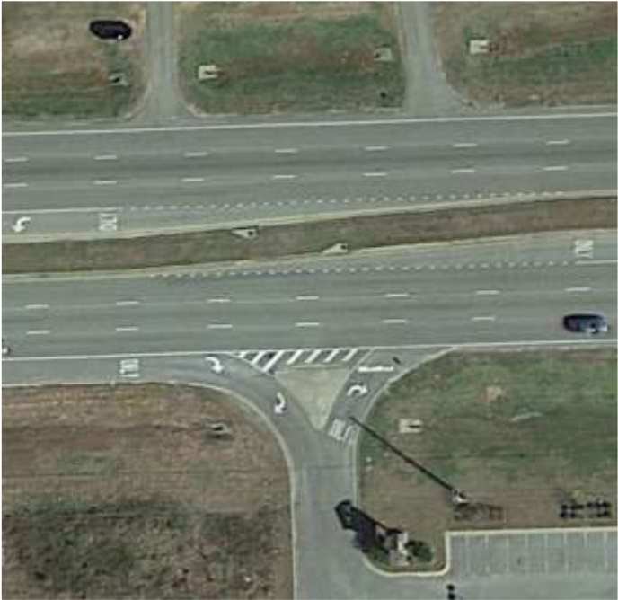
Right In / Right Out - Limiting Street and/or Driveway Entrances to "Right In / Right Out"
