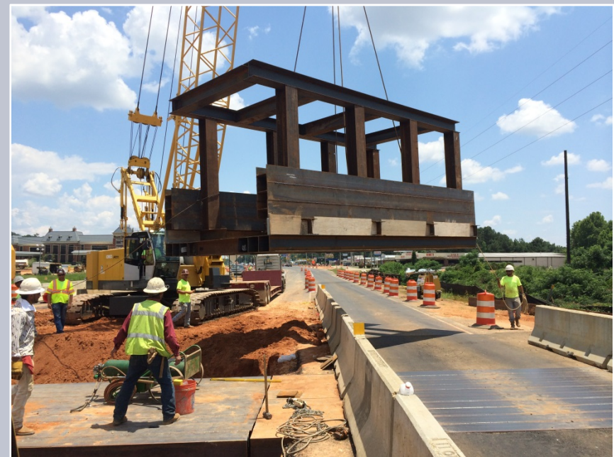
Shoring boxes being erected and set in the trench.
