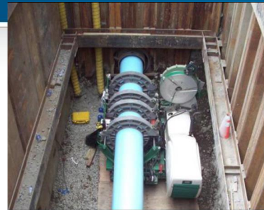
Anchorage, AK: 24" DR18 in 30" Steel Casing
