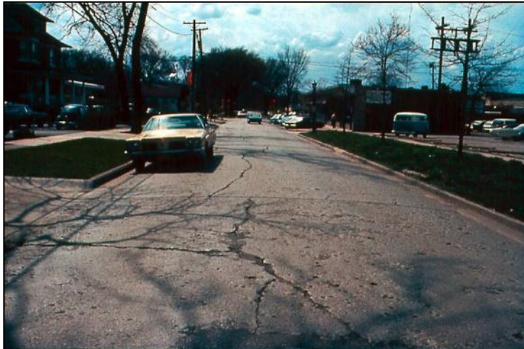
Erratic crack patterns due to no joints
